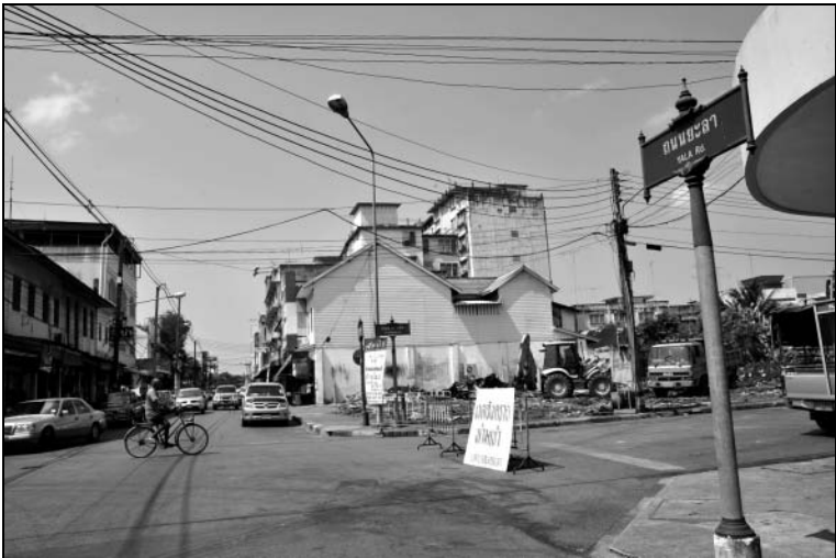
A block of shop houses totally destroyed by a car bomb attack in Yala city market in March 2011 (Photo François May, March 2011)
